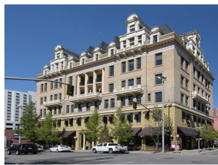
The grand American Legion Building was one of the first structures in Spokane to be built with fireproof structural steel and have high speed electric elevators.
